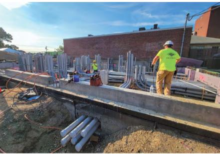
Restoration of Brockton Hospital after a February 2023 fire employed as many as 60 IBEW electricians a day from Brockton, Mass., Local 223, and Boston Local 103. A vast list of projects included installing underground pipes, pictured above, for a new exterior electrical room, and, at bottom right, more pipework feeding the hospital itself. At top right is a section of wiring for 3,000 solar panels that members installed above carports in the parking lot.
